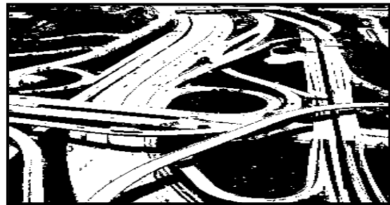
Figure 11.2.1.9c: Risky freeway and traffic systems
