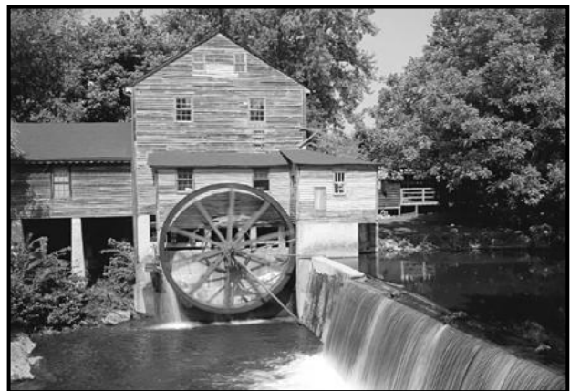
Figure 11.2.1.8b: Water Powered Mill
